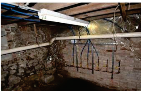
New copper + pex plumbing.
